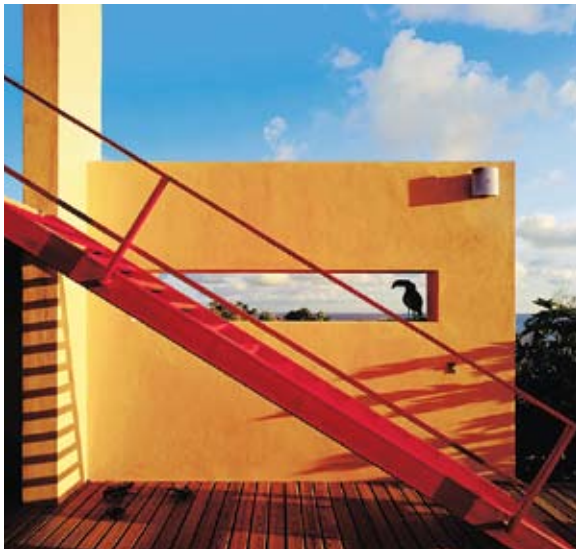
The Taylor vacation house looks out on the Sea of Abaco in the Bahamas. It's sheltered from the intense summer sun by an inverted umbrella roof that also collects rainwater for all
